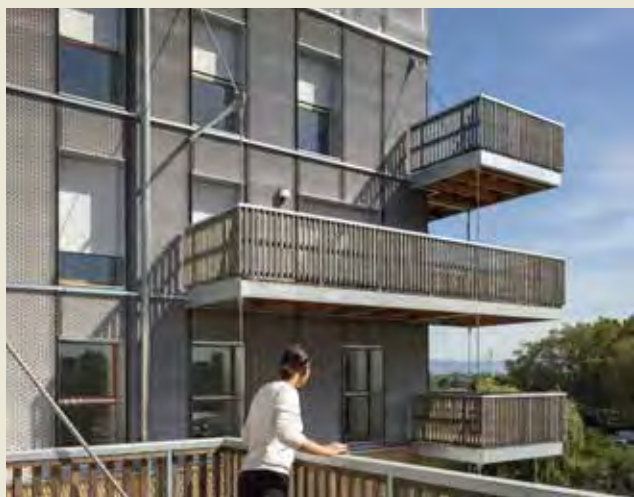
© Cécile Septet, KOZ Architectes, ASP Architecture, Bouygues Immobilier
